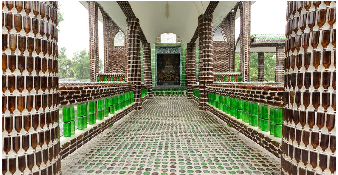
Recycle building materials
